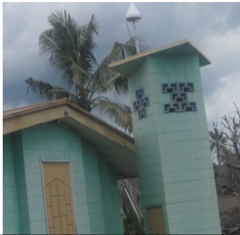
Figure 3. Remote GPS station (SDA) antenna on the roof of a church building on Matupit Island.
